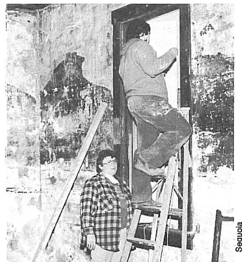
Renovation in progress at the new Crazy Ladies.
